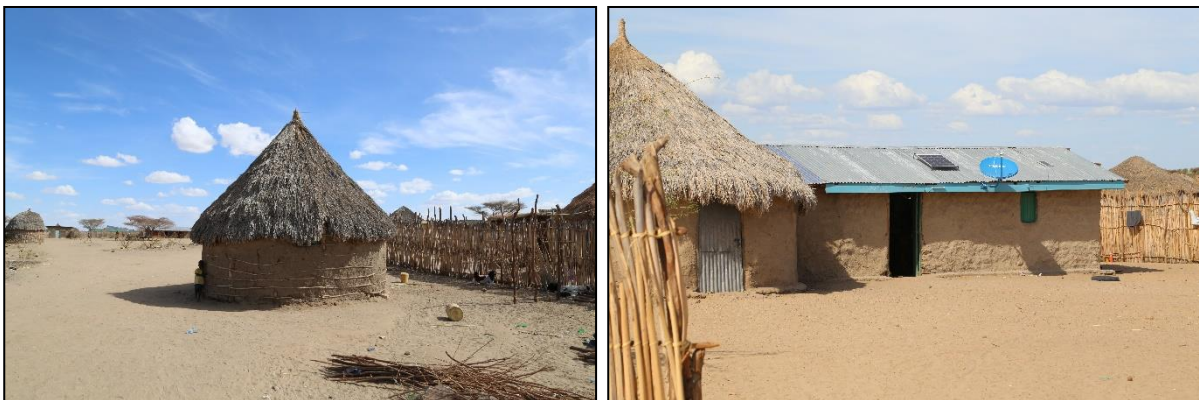
Fig.4.2 – Traditional semi-permanent building, normally a household (left) and image of a permanent structure made from timber, cladding and iron sheets, normally containing a business (right).
